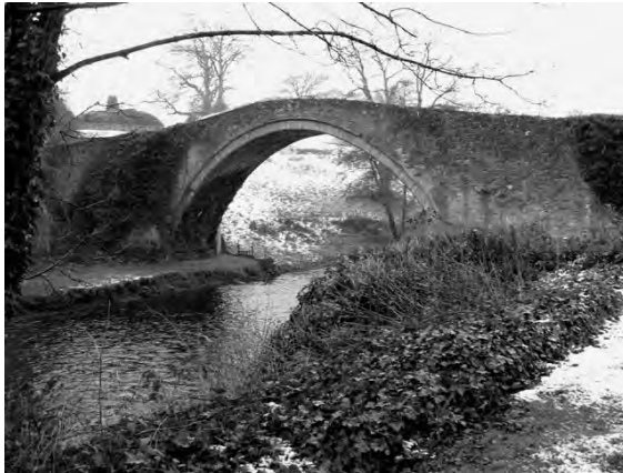
1. Bridge over the Doon River/Ayrshire, Scotland
